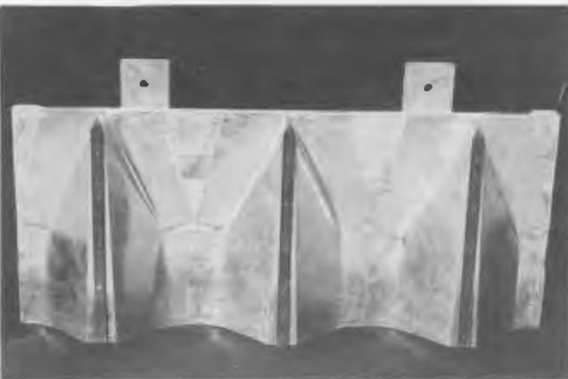
**Photo 7. Note strap iron attachment and sheet metal attachment to under surface of platform.**
