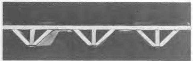
**Photo 8. Note trailing edge of sheet metal shaped in an arc to form rounded ridge tops.**
